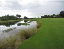
m. Lake 58 – A large washout has developed between 9230 & 9236 Gypsum Way. The lake bank should be repaired quickly before the issues gets more severe. Drainage from the adjacent structures should likely be piped directly into the lake below the low-water mark to prevent further erosion.
