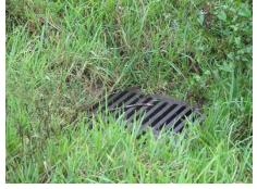
ii. W1L30: The control structure was not flowing. The torpedo grass and all weeds should be sprayed out. There was at least one section of concrete dislodged that should likely be repaired.
