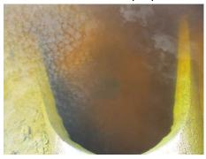
2. A piece of wood was found in a junction box behind 9070 Limestone Ln. that should be removed to prevent a possible blockage.
