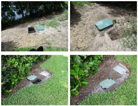
b. After a heavy afternoon rain, water could be heard flowing next to the restrooms along conservation area #2, but no drain was visible. The drain was uncovered and the water was able to drain more quickly in the area.
