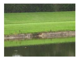
ii. A washout is occurring on the eastern bank between the tee boxes of the #13 hole and the heavy downpours appear to be overflowing attempts to control the water flow. A flume may be considered in this area or a drain to be installed on the cart path with piping into the lake below the low-water mark.
