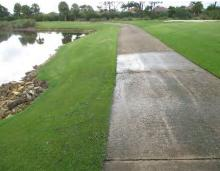
j. Lake 45 – erosion is occurring on the northeastern bank. Drainage from the adjacent structures should be reviewed and piping installed to direct the water into the lake below the low-water mark.
