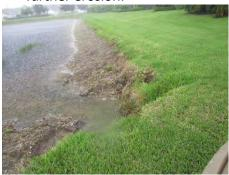
n. Lake 61 – There is a large washout between the homes of 9020 & 9024 Graphite Circle. It is recommended that the downspouts of these homes be connected to drainage that is ran directly into the lake below the low water mark to eliminate the erosion issue.
