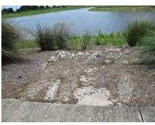
iv. There are three areas on the west bank of lake 30 that are being eroded along the #18 hole that line up with fairway drains. If there is not a maintenance plan to manage drains and ensure they are clear before and after heavy rains events one should be encouraged to be implemented to help minimize such erosion. If a drain maintenance program is in place, consideration of larger drains or those with larger openings may need to be considered.
