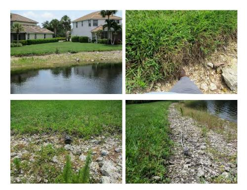
viii. The pool overflow for 9167 Shale Ct. has been rerouted to discharge directly into the lake and as a result minimal erosion is occurring on the south bank of lake 38, but more importantly due to the discharge directly occurring on the lake bank littorals in this area will be impacted and likely prohibited from developing. The pool overflow should be corrected and installed per County requirements. Additional comments noted under the Illicit Discharge section of the report.
