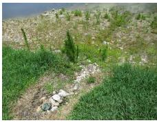
ii. Step erosion was observed on the northwest bank of lake 36 that should be monitored.
