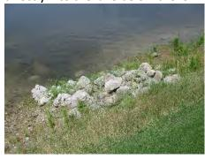
c. Lake 35 – Step erosion is occurring on the south bank that will need to be addressed in the future. Drainage from the adjacent structures should be reviewed to see if they are contributing to the erosion.
