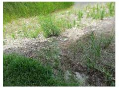
e. Lake 37 – Irrigation has been placed on the north bank below the high-water mark and should likely be relocated to avoid erosion of the bank. Additionally, there is a large hole in the west bank of the lake that should be filled before a larger issue develops.
