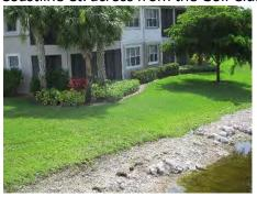
iii. Erosion is beginning to develop on the southeast portion of lake 30 adjacent to the tee boxes for hole #18. Installation of curbing may be considered or the addition of a drain at the cart path low point to minimize lake bank erosion in the area. It appears that golf course plugs have previously been added on the west side of the cart path for the same issue.
