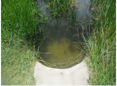
iii. 38: The roadway drain discharge pipe appears not to be level presently. It is possible the pipe was set initially at an angle. The pipe should be monitored to see if further movement is visible.
