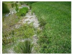
ii. Erosion is developing between the homes of 9115 & 9119 Crystal Ct. The Board may wish to consider having drainage added in the area to minimize further erosion from developing.
