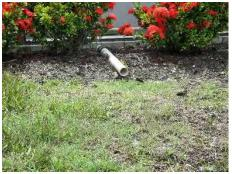
vi. 9298 Quarry Dr.: It appears a pool overflow drain has been rerouted from the home to the northwestern swale catch basin which flows directly to lakes 57 & 58. The discharge into the catch basin should be removed.
